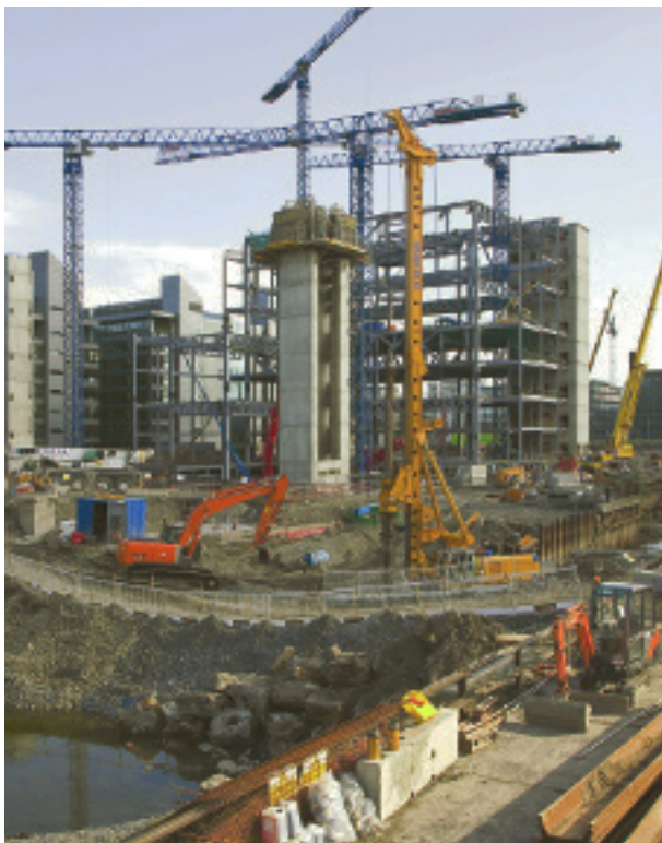
Transport 21 is transforming Ireland's transport infrastructure at a total cost of €34 billion
