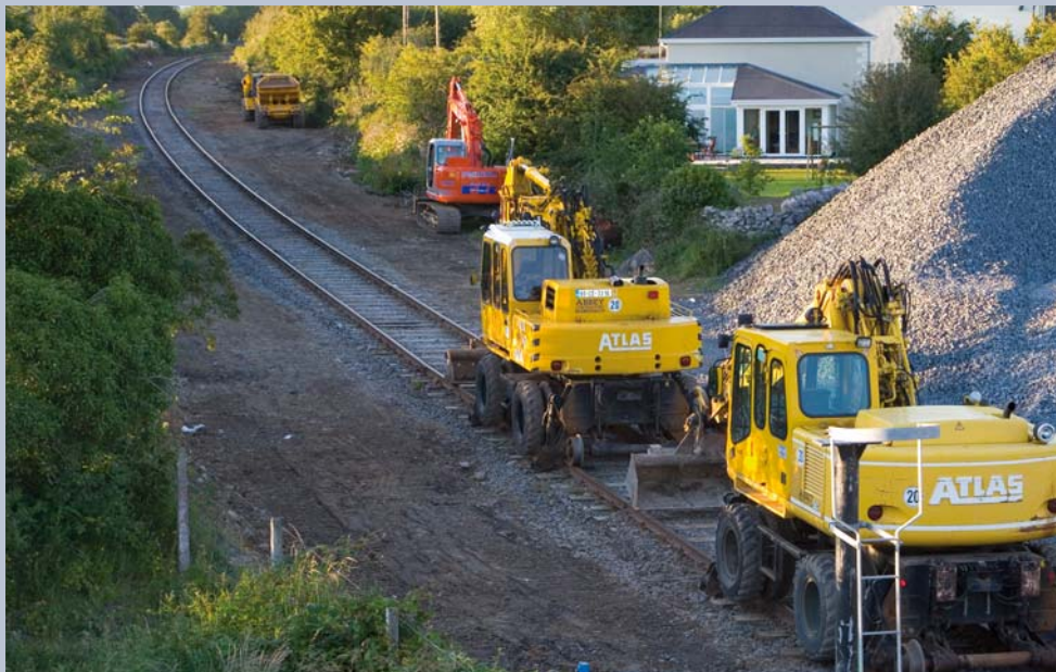
Work on the Western Rail Corridor
