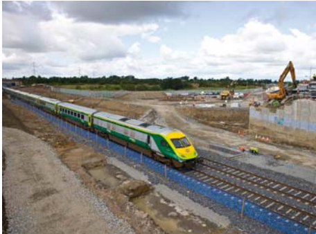
Ongoing work on the Kildare Route Project
